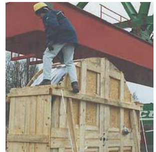
■ Assembly of the fully harnessed cable carrier system
